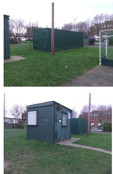
C305 Site Photos of existing shed and container
